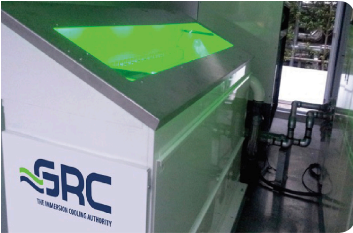
Fig. 4. The GRC ICERaQ system installed inside the module
