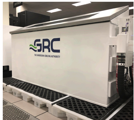
ICEraQ system's secondary containment decks catch any accidental coolant spills and keep data centers tidy.
