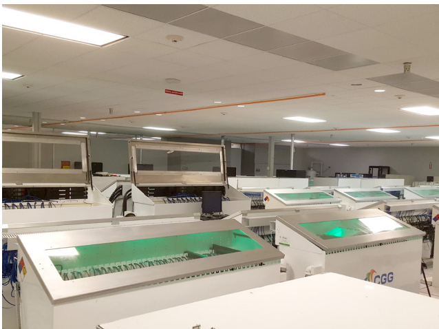
Image 1: GRC's immersion-cooled ICEraQ® systems provide an open, quiet, comfortable work and data environment..
